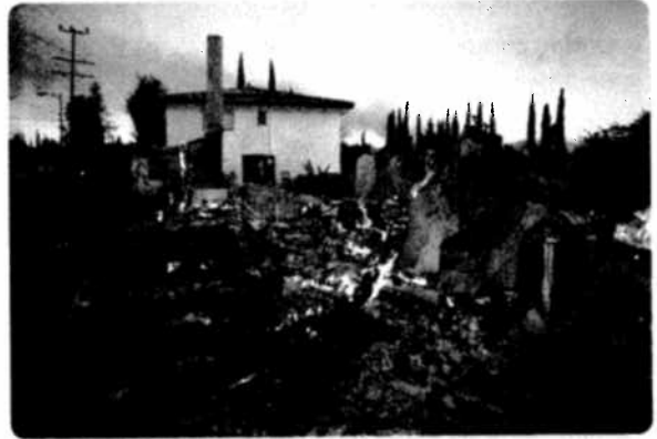
FIRE Many fires broke out after the Northridge, California, earthquake in 1994.
