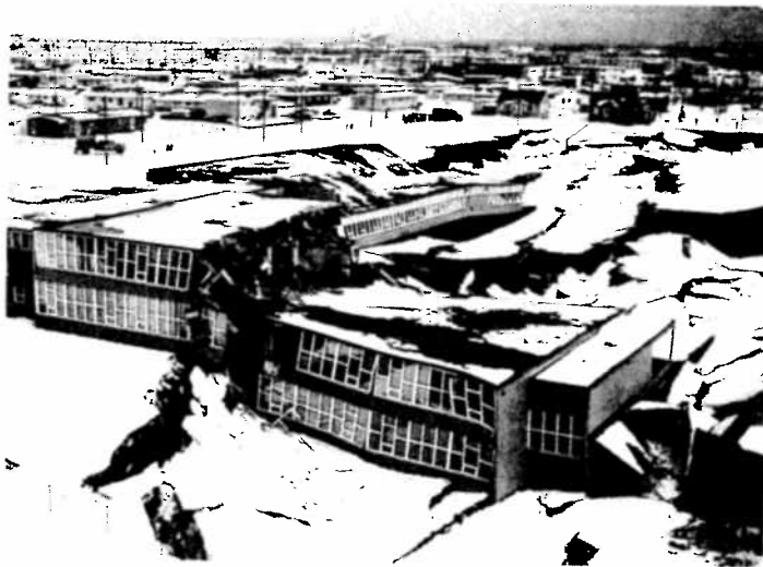
ALASKA, 1964 The earthquake that struck along the coast of Prince William Sound in 1964 caused massive displacements along faults.
