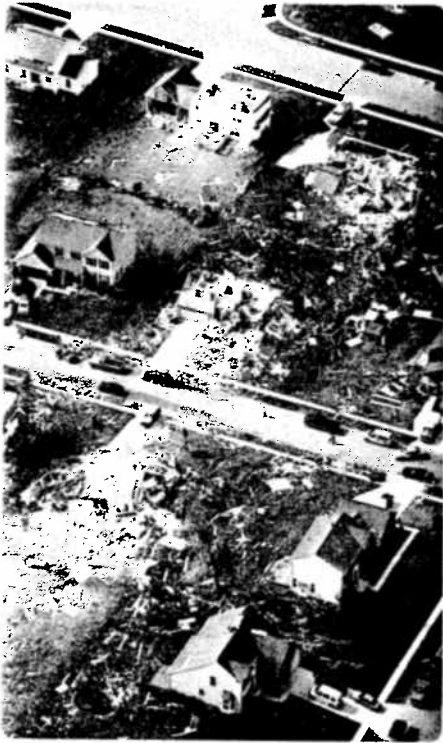
TORNADO DAMAGE Because a tornado can be only meters across, it can destroy some buildings completely while leaving structures next door virtually untouched.
