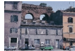
Above: An aqueduct approaching Rome. It carries two water channels, one above the other.
