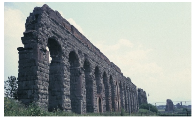
Above: An aqueduct approaching Rome. It carries two water channels, one above the other.
