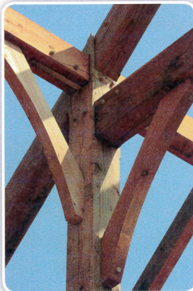
Figure 1-13: Mortise-and-tenon joints were used in this wooden post-and-beam construction.
