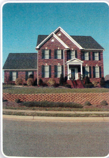
Figure 1-6: The retaining wall in the foreground of this photo must withstand pressure from the lateral movement of the earth behind it and stormwater runoff.
