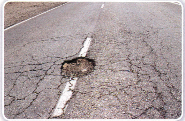
Figure 1-51: Road cracks and pothole.
