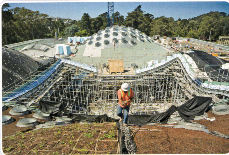
Figure 2-11: Academy of Sciences building in Golden Gate Park, San Francisco, California is a LEED-certified building with a living roof and photovoltaic panels.
