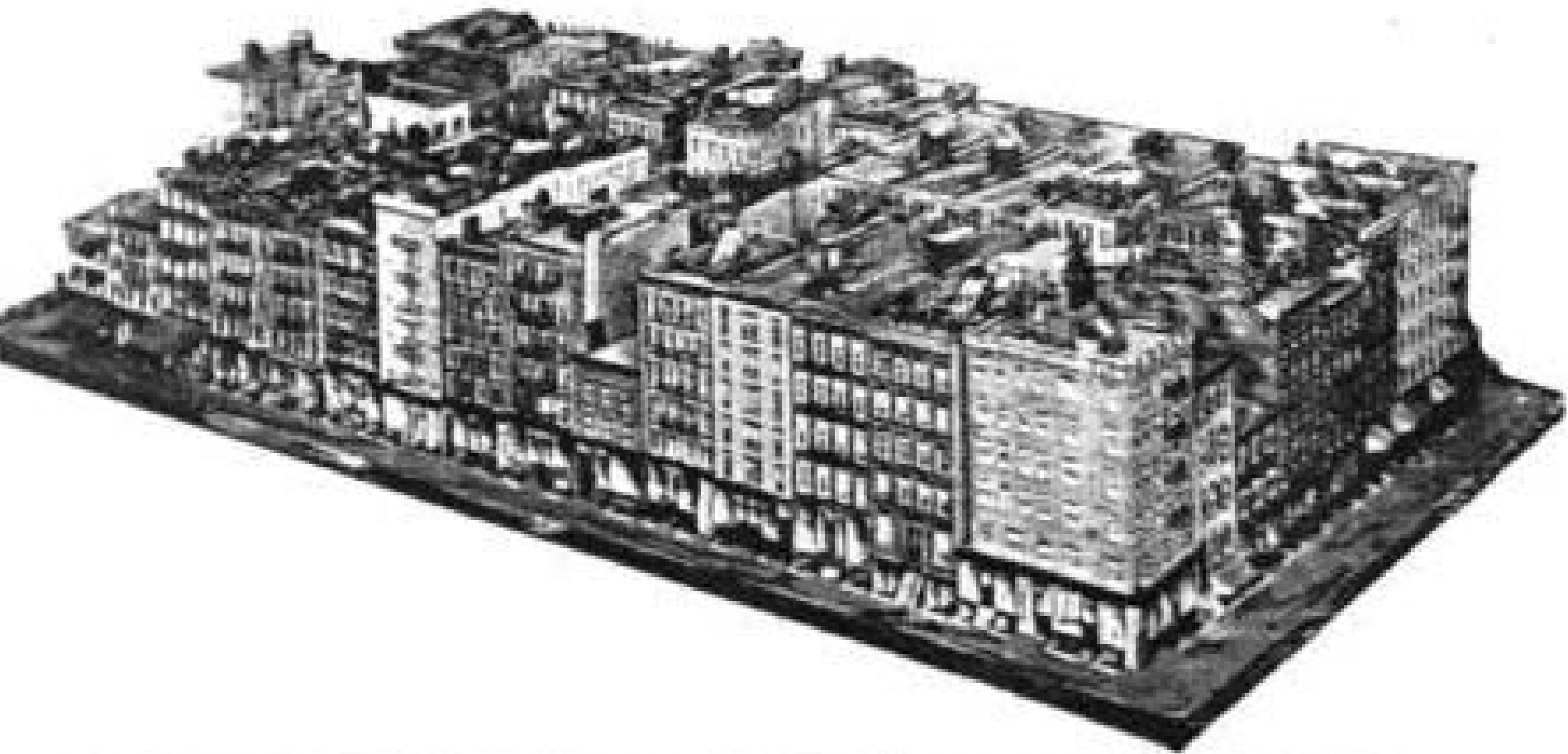
AN EXISTING BLOCK OF TENEMENTS IN 1900 ON THE LOWER EAST SIDE OF NEW YORK.
