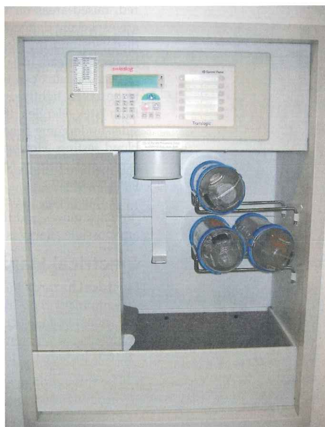
Figure 2-4 Vacuum system pneumatic tube station. Sandra Mesrine/McGraw-Hill Education
